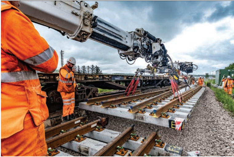
● Aberdeen Inverness double- tracking works
